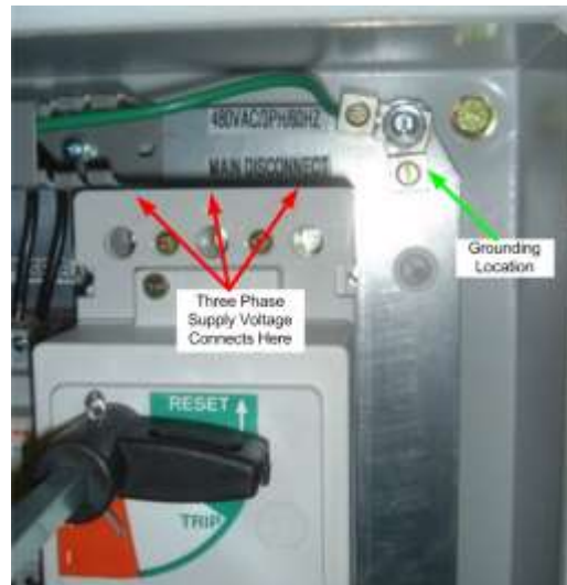
Supply Voltage Termination Points (480VAC shown)
